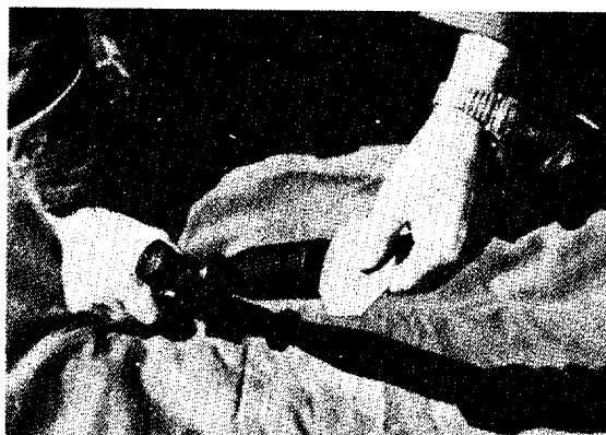
Figure 2-6. Adjusting Parallax With "Spanner."
